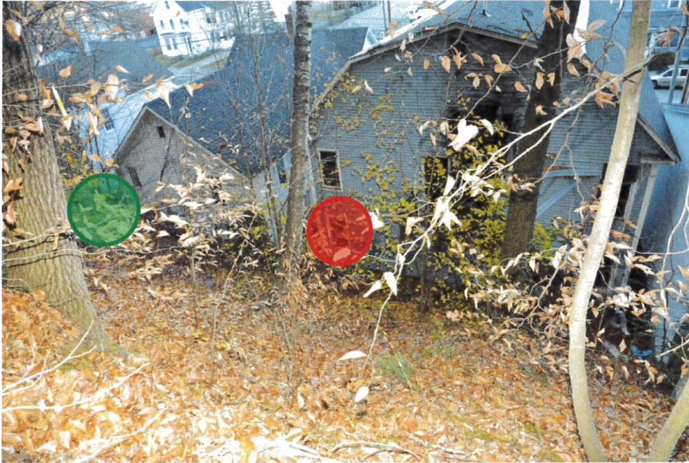
A photograph of the rear 32 West Bow Street taken from the approximate position of Troopers Caraballo and Powers in the steeply-sloped wooded area behind the building. The window highlighted in red is where Mr. Landrebe was when he discharged his shotgun outwards, and the area highlighted in green is Trooper Wong-Wagner's approximate location at the time.
